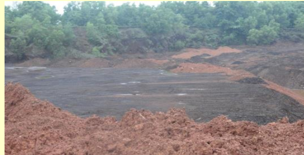
Back filling of exhausted pits
